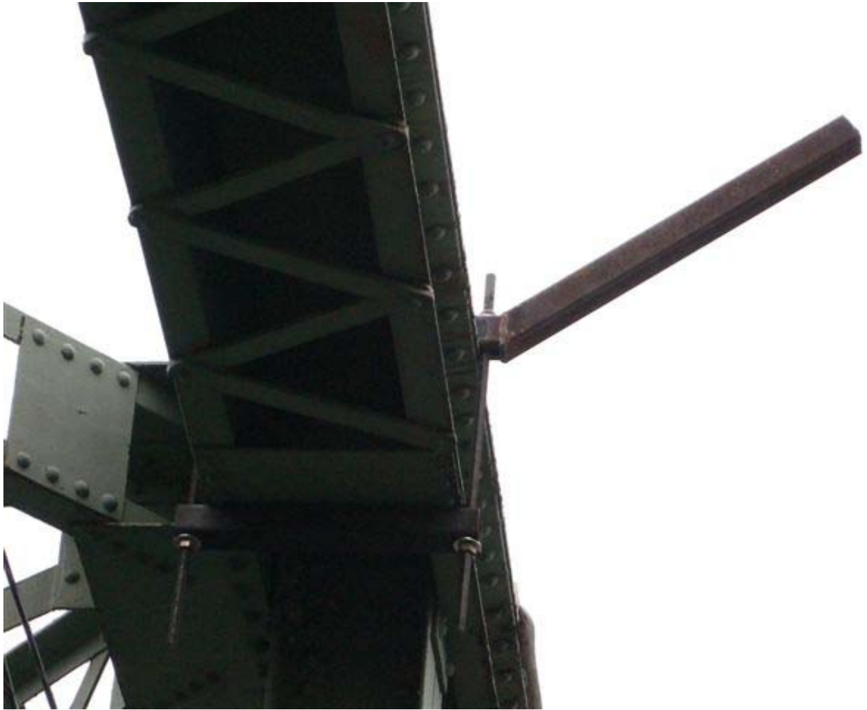
Upper Level Containment Brackets
