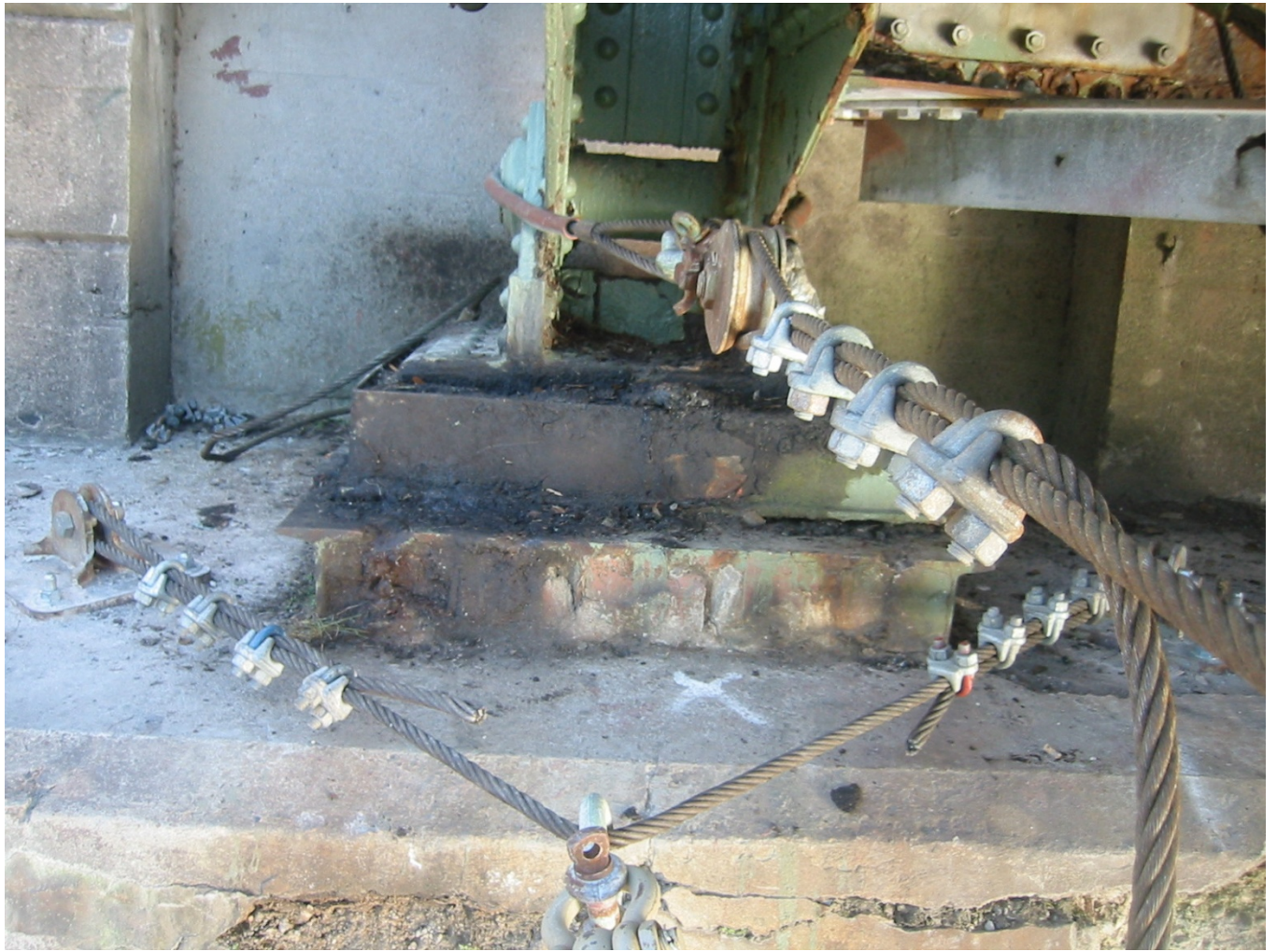
Anchor Plate End Connections-Inner Cables
