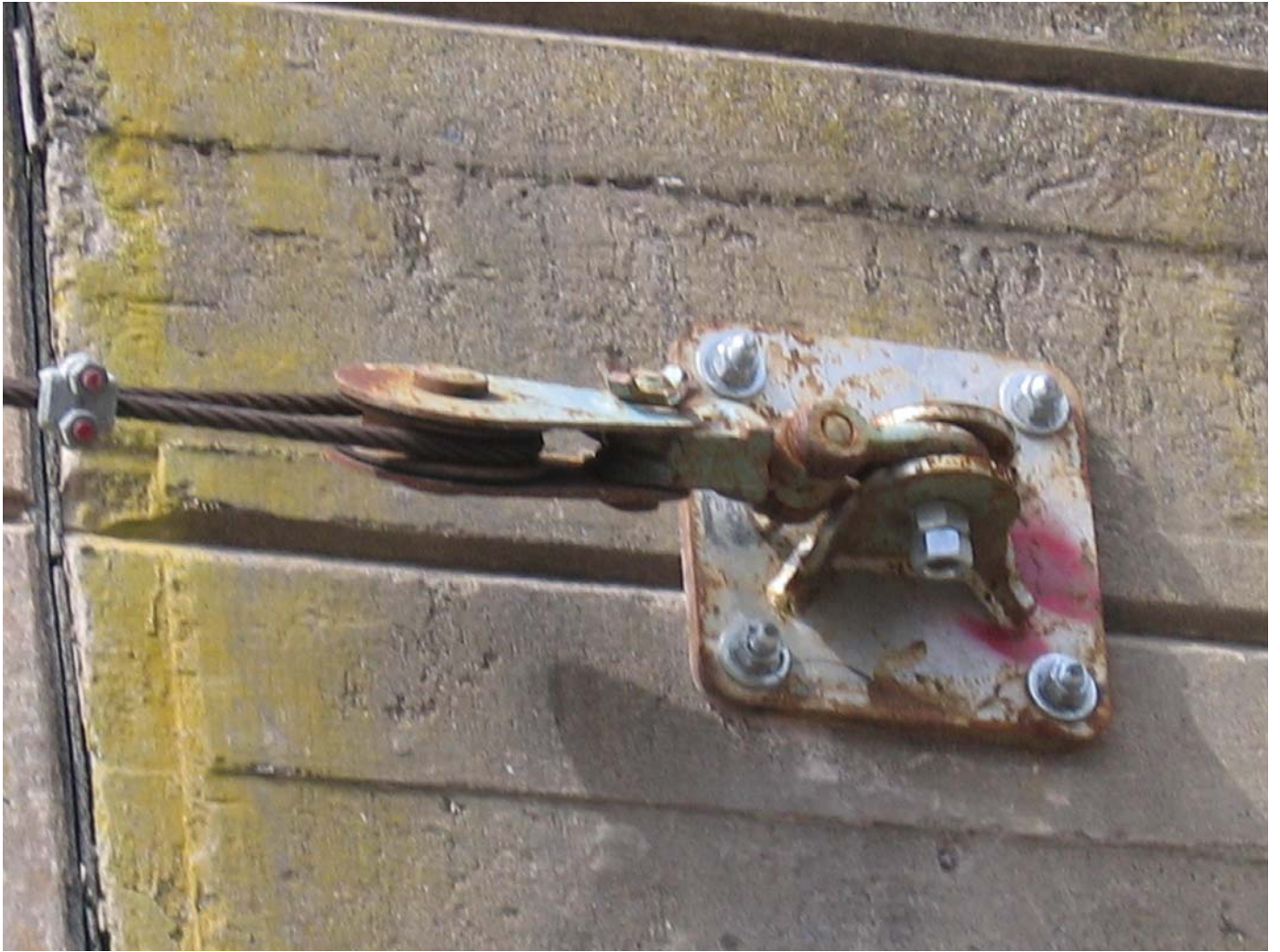
Anchor Plate End Connections-Outer Cable
