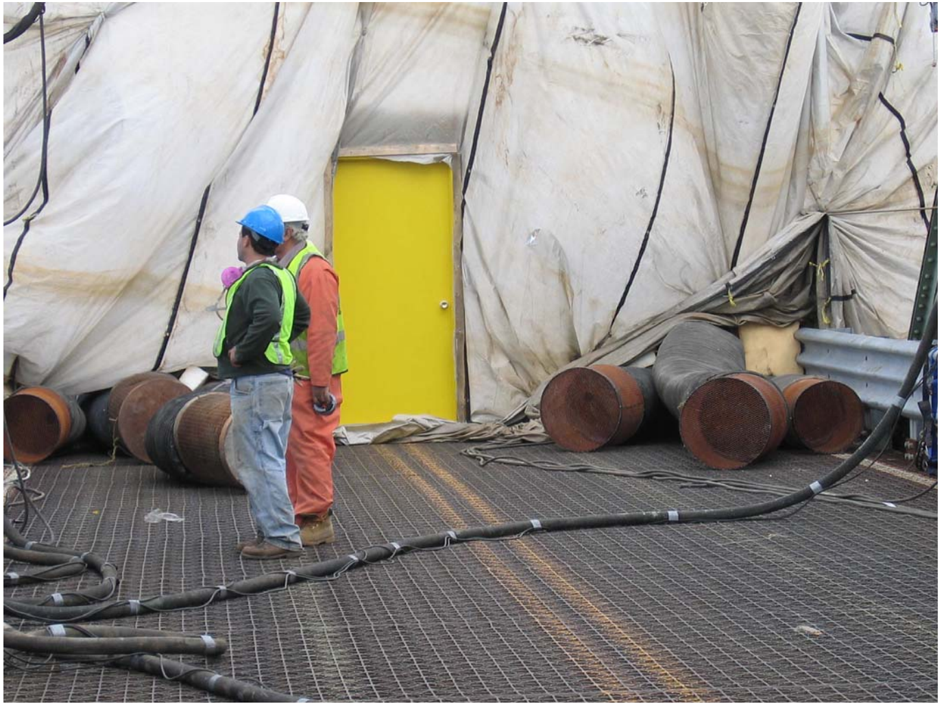
End Containment & Entry Air Lock
