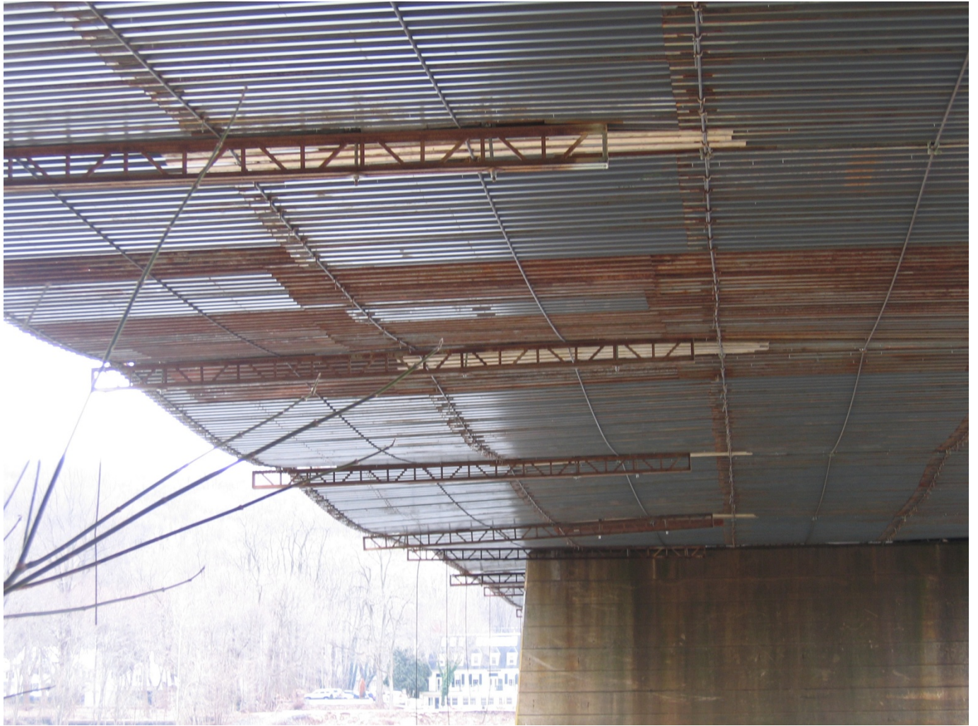
Main Cable Tie Up Support Trusses
